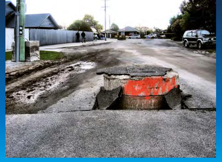
Sewer lines floats in liquefaction area pushing manholes up
