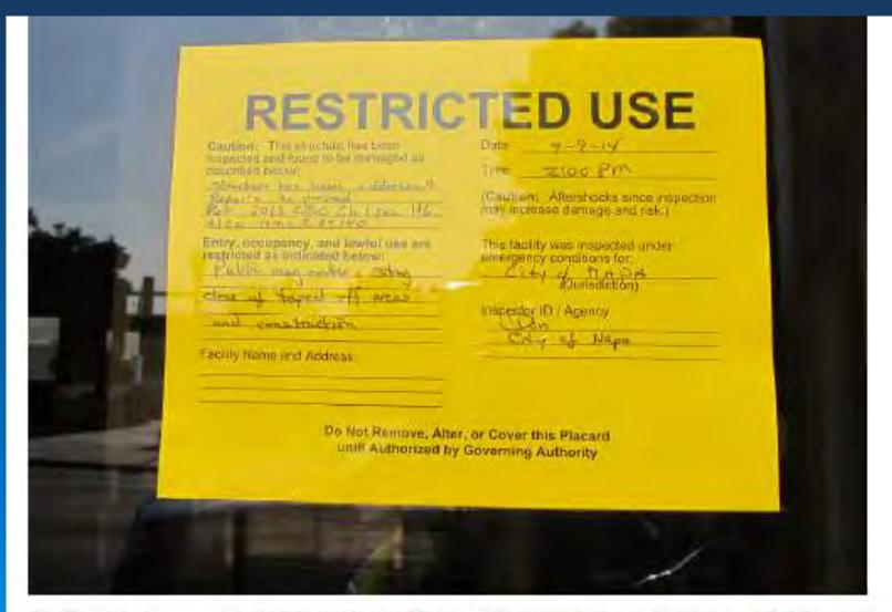
Figure 11-2 A RESTRICTED USE tag with restrictions noted as "Public may enter. Stay clear of taped off areas and construction."
